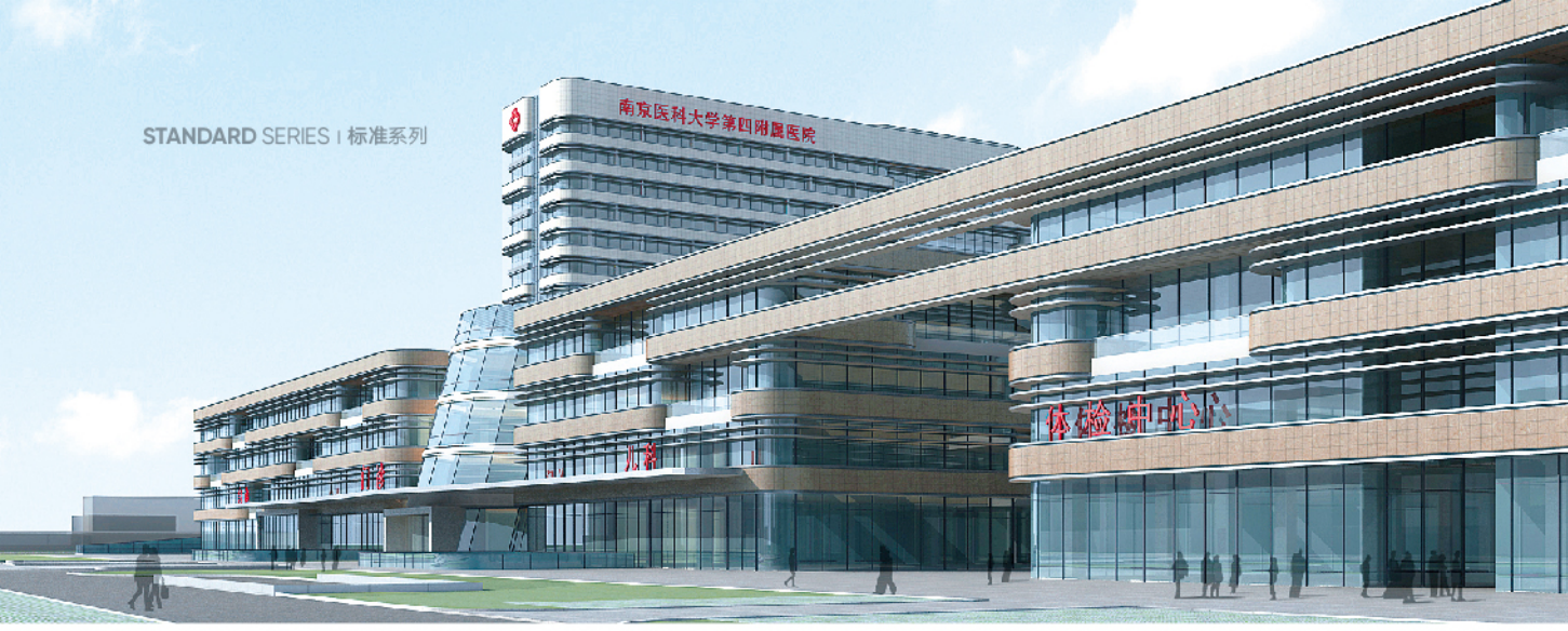
南京医科大学第四附属医院 A级不燃铝复合板40000m 2 The Fourth Affiliated Hospital Of Nanjing Medical University Class A FR ACP 40000m 2
