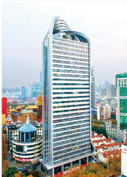
上海静安中华大厦 飞腾铝复合板25000m 2 Shanghai Jingan Zhonghua Building ACP 25000m 2
